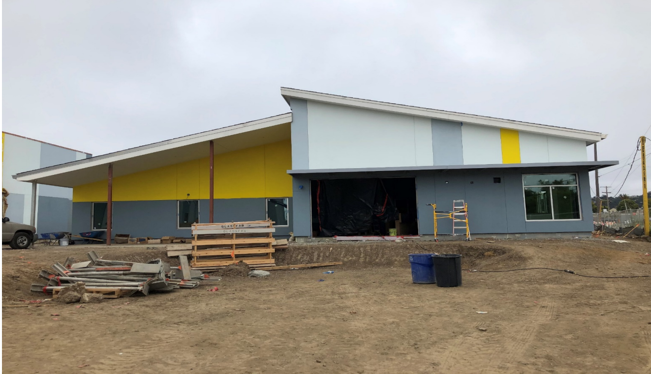
Administration Entry with Canopy
