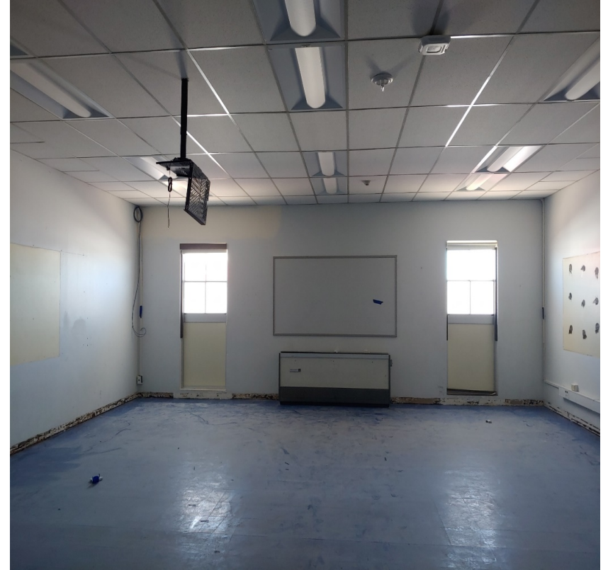
Science Building Ceiling Replaced
