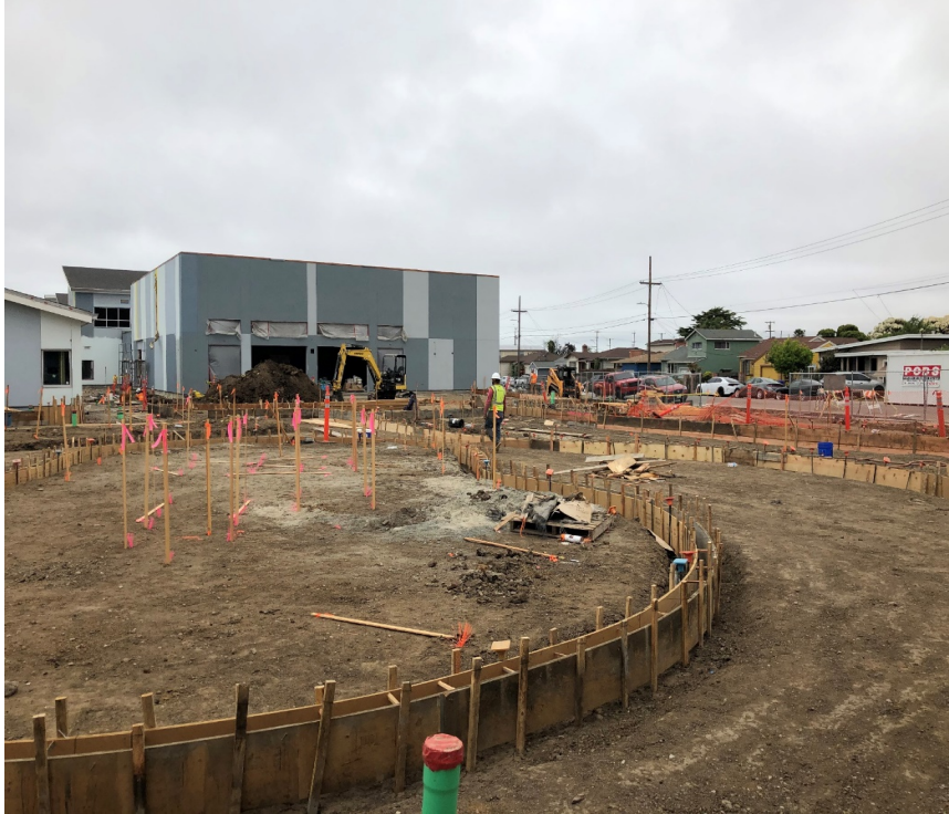
Kindergarten Play Area Formwork
